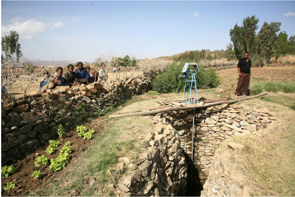
Figure 4: Rope pump lifting water from a dugwell in Ethiopia. Photo: MetaMeta.
