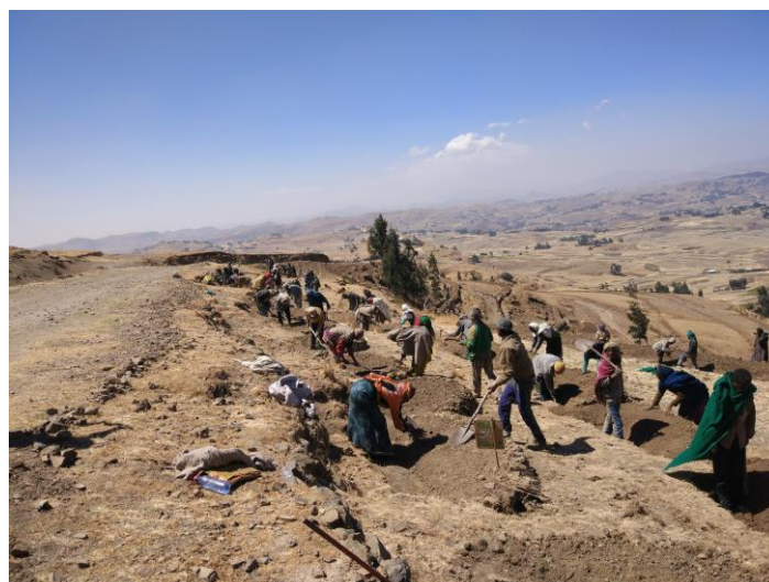
Figure 2: Groundwater recharge at scale: making half-moons to harvest road water in Ethiopia. Photo: MetaMeta.
