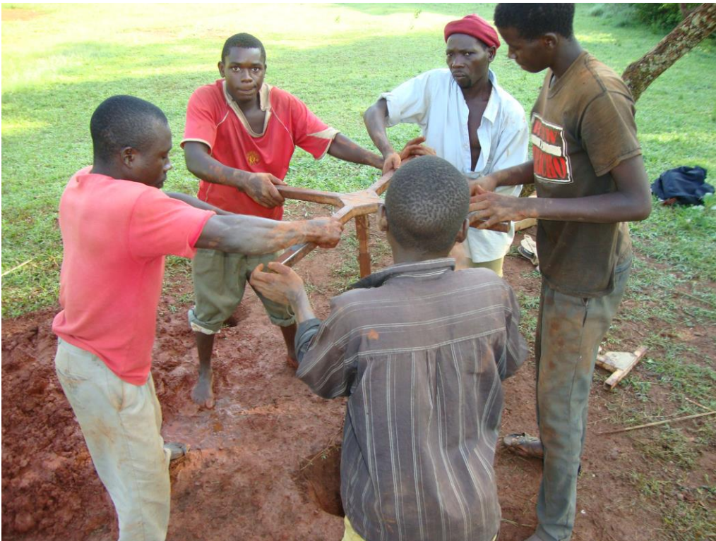
Figure 3: Developing new well by manual augering in Uganda. Photo: MetaMeta.
